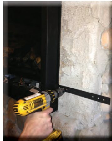
2. Screw the template to framing using the appropriate fastener.
