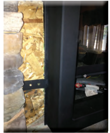
2. Screw the template to framing using the appropriate fastener.
