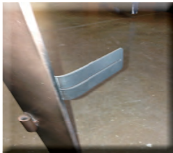
4. Bend the welded tabs on the door frame inward.
