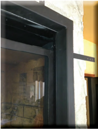
1. Square template to top & bottom on the DV unit.
