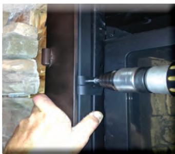
6. Pre-drill a pilot hole through welded tab and through the DV template. Install screw through welded tabs and into the DV template securing the door.
