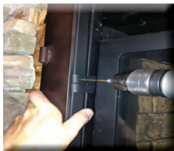
6. Pre-drill a pilot hole through welded tab and through the DV template. Install screw through welded tabs and into the DV template securing the door.
