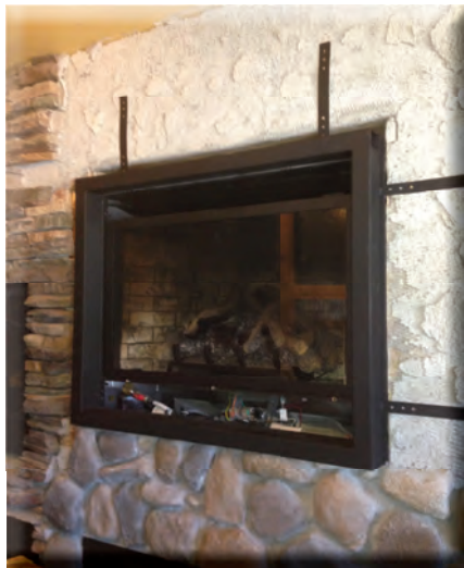
3. Template is attached to the framing and is ready to be rocked in, then receive the door.
