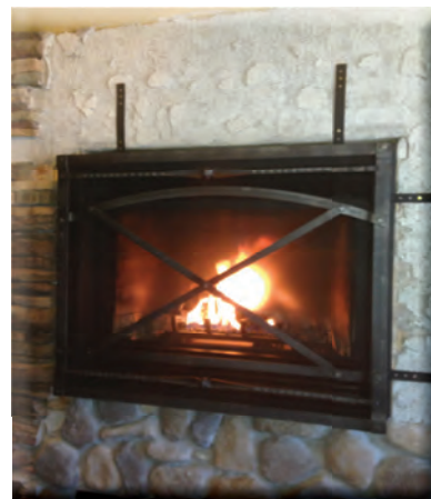
5. Measure the distance that you have for the welded tabs to go inward on the DV unit / DV template, (in this case we have 2”).
