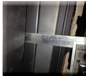
5. Measure the distance that you have for the welded tabs to go inward on the DV unit / DV template, (in this case we have 2”).
