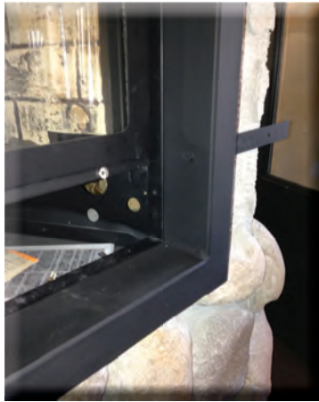
1. Square template to top & bottom on the DV unit.
