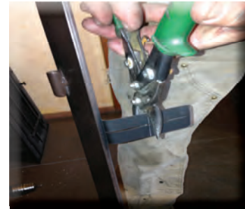
3. Trim the welded tabs, if needed to the measured length..
