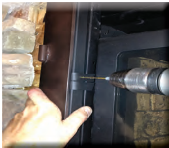
4. Predrill a pilot hole through welded tab and through the unit. Install screw through welded tabs and into the unit securing the frame to the unit.
