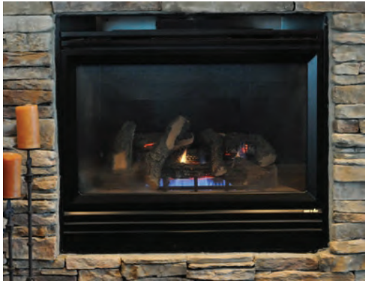
Direct vent gas fireplace before mounting a Lifestyle Series or Heritage Series door.
