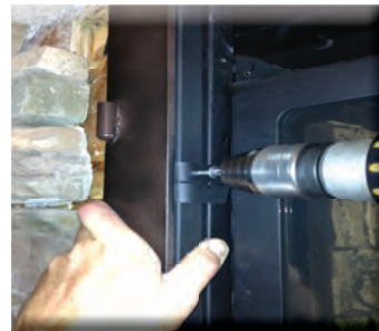
4. Predrill a pilot hole through welded tab and through the unit. Install screw through welded tabs and into the unit securing the frame to the unit.
