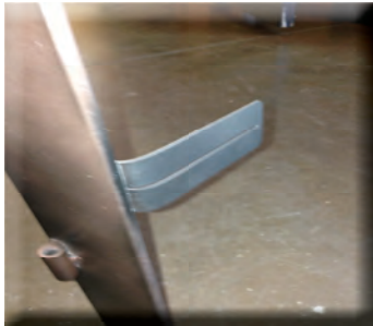
1. Bend the welded tabs on the door frame inward.
